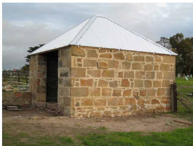
Roof completed but awaiting gutters. Photography: Dr Rob Sloane.
