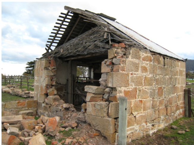
The building before work commenced. Photography: Dr Rob Sloane.
