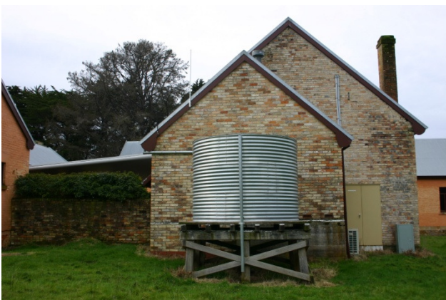
Appropriately installed water tanks at the Asylum Building, Port Arthur, Photography: Port Arthur Historic Site
