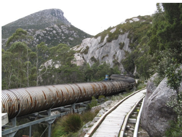
Lake Margaret woodstave pipeline. Photography: David Scott
