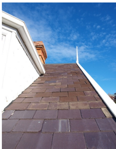
The new slate roof. Photo: Robyn Shaw
